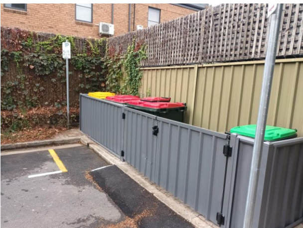
Image: After bin surround installation
