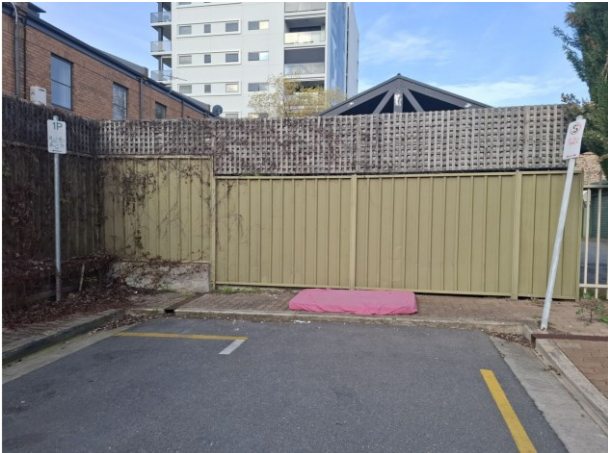
Image: Before bin surround installation
